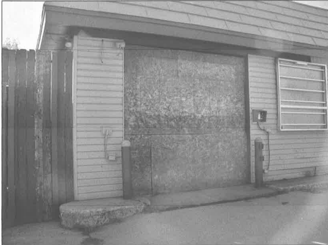
5720 N. Oak Trafficway – looking west – deterioration of door, siding, signage; failure of finishes
