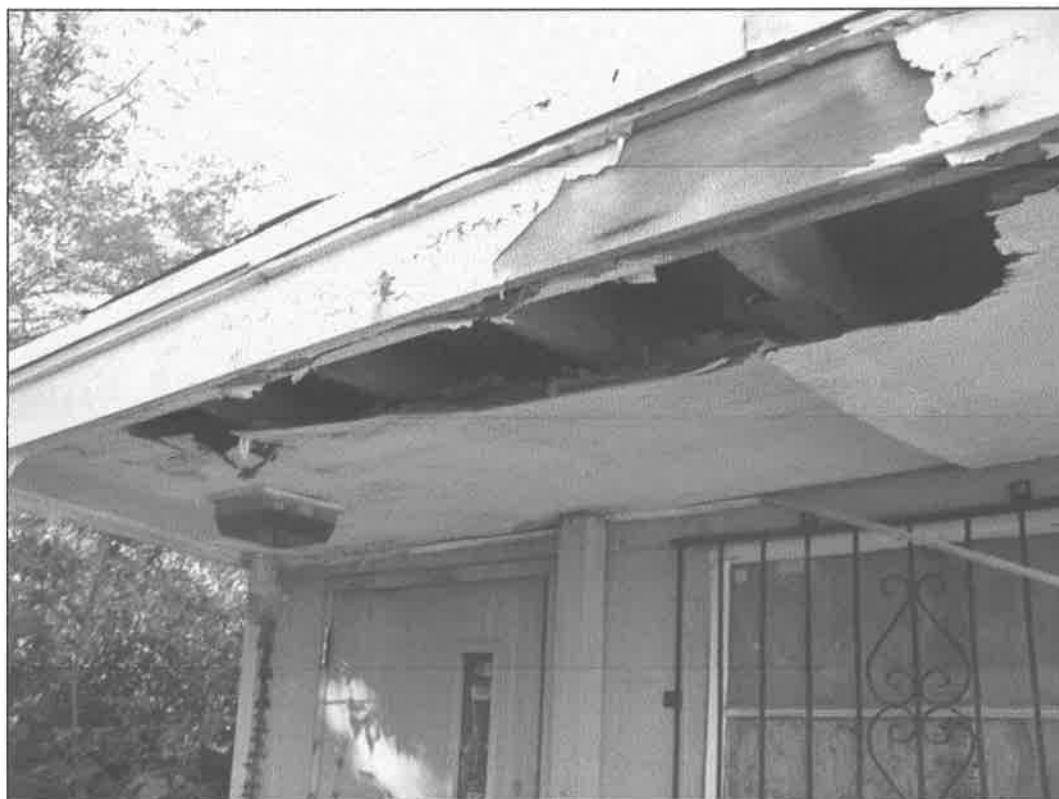
307 NE 58 th Street – looking north – deterioration of fascia, soffit, window, roof coping; failure of finishes
