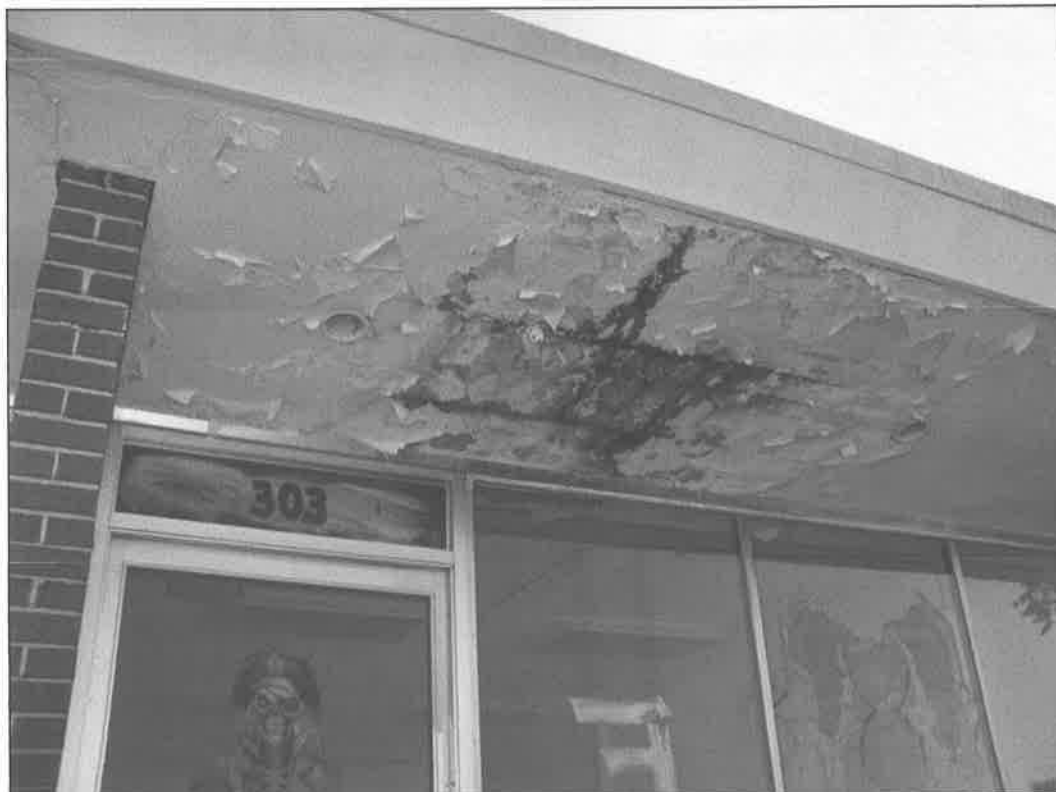
307 NE 58 th Street – looking south – deterioration of soffit (due to leaking roof)
