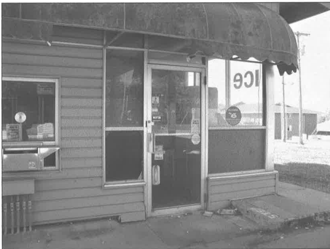
5720 N. Oak Trafficway – looking northwest – deterioration of awning, sidewalk; failure of finishes
