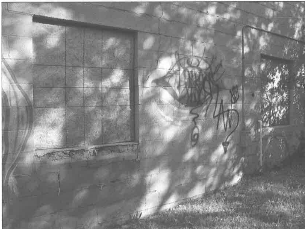
307 NE 58 th Street – looking east – cracked and spalling masonry wall; deterioration of window; failed finishes
