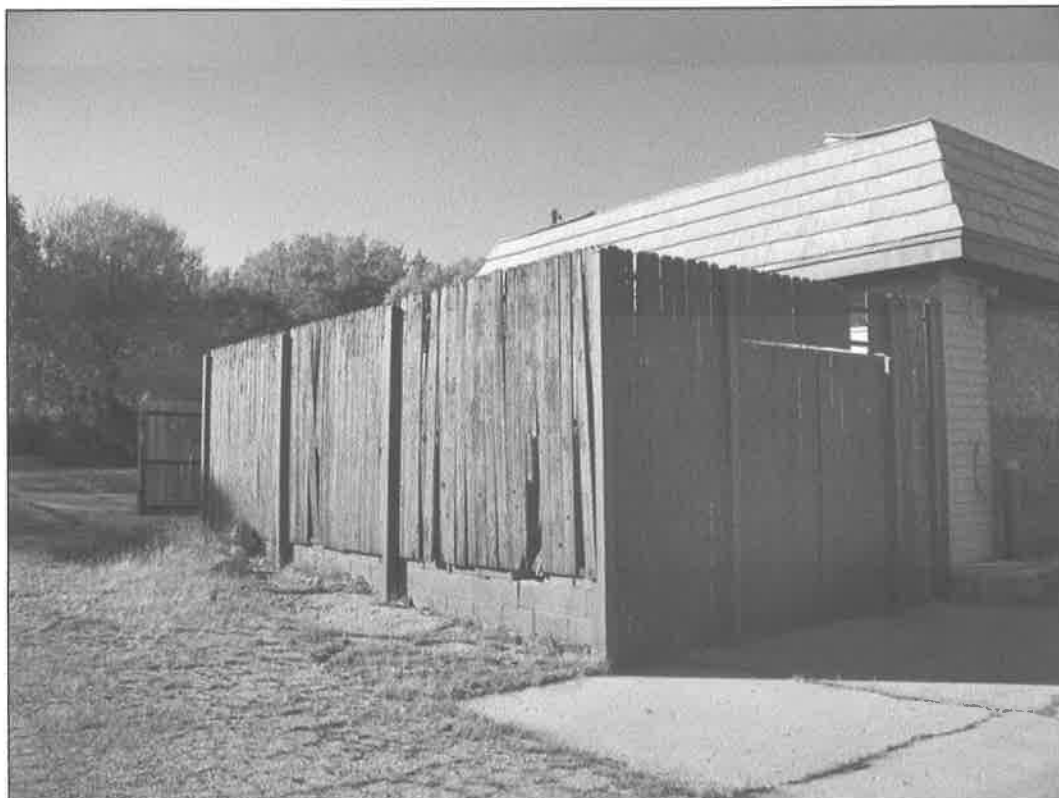
5720 N. Oak Trafficway – looking northwest – deterioration of fence, masonry wall, driveway
