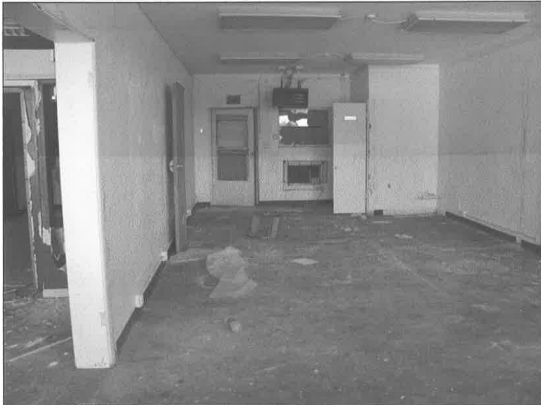
307 NE 58 th Street – looking south – deterioration of interior finishes, windows, doors; outdated building systems
