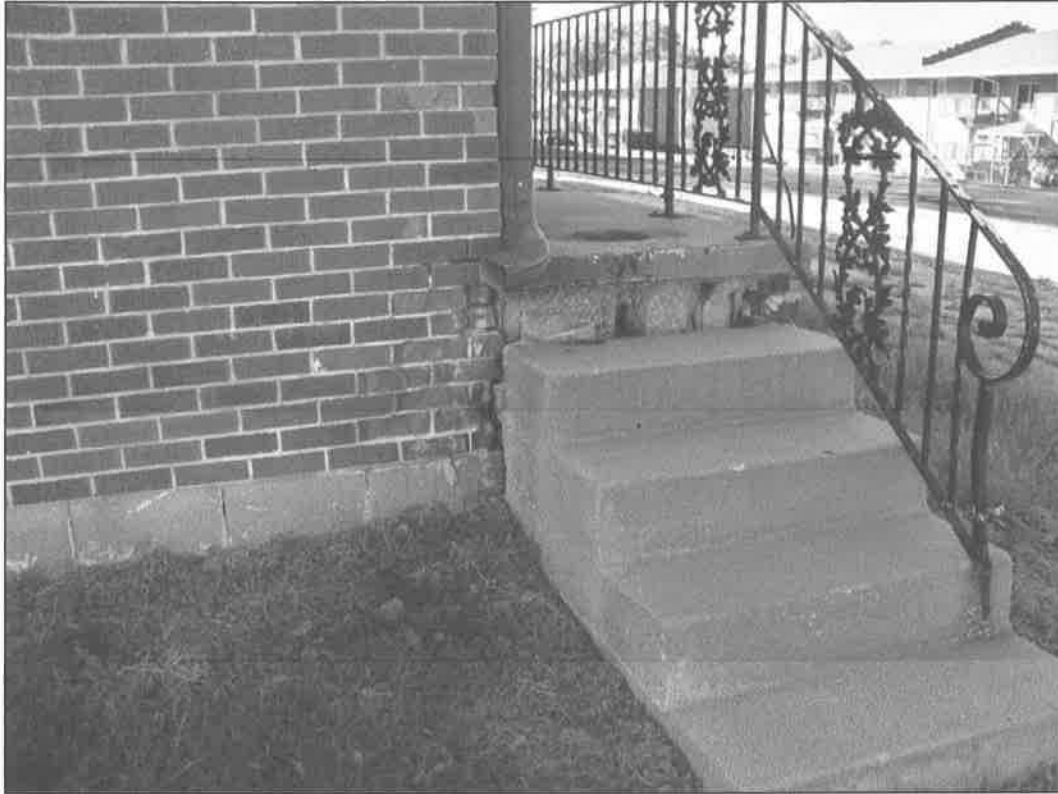
307 NE 58 th Street – looking west – deterioration of masonry veneer, steps; failure of finishes
