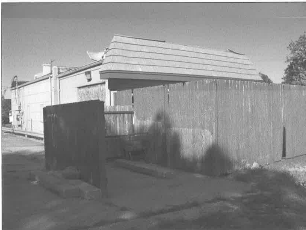
5720 N. Oak Trafficway – looking northeast – failure of finishes; deterioration of fence, driveway
