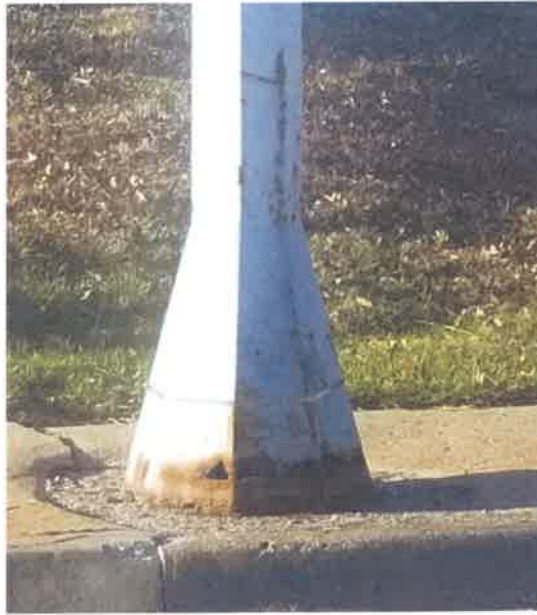
NE 72 nd Street & N. Troost Avenue – Traffic Signal Base (Prior to Temporary Repair)
