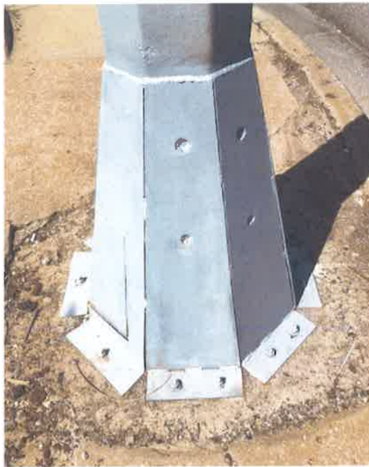
NE 72 nd Street & N. Troost Avenue – Traffic Signal Base (After Temporary Repair)
