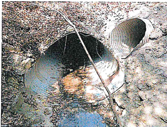
CMP Culvert Outlet at 6809 N Agnes Avenue
