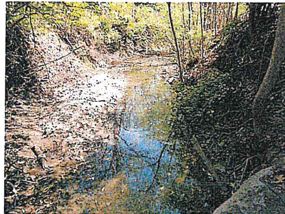
Typical Bank Erosion at 6709 N Agnes Avenue
