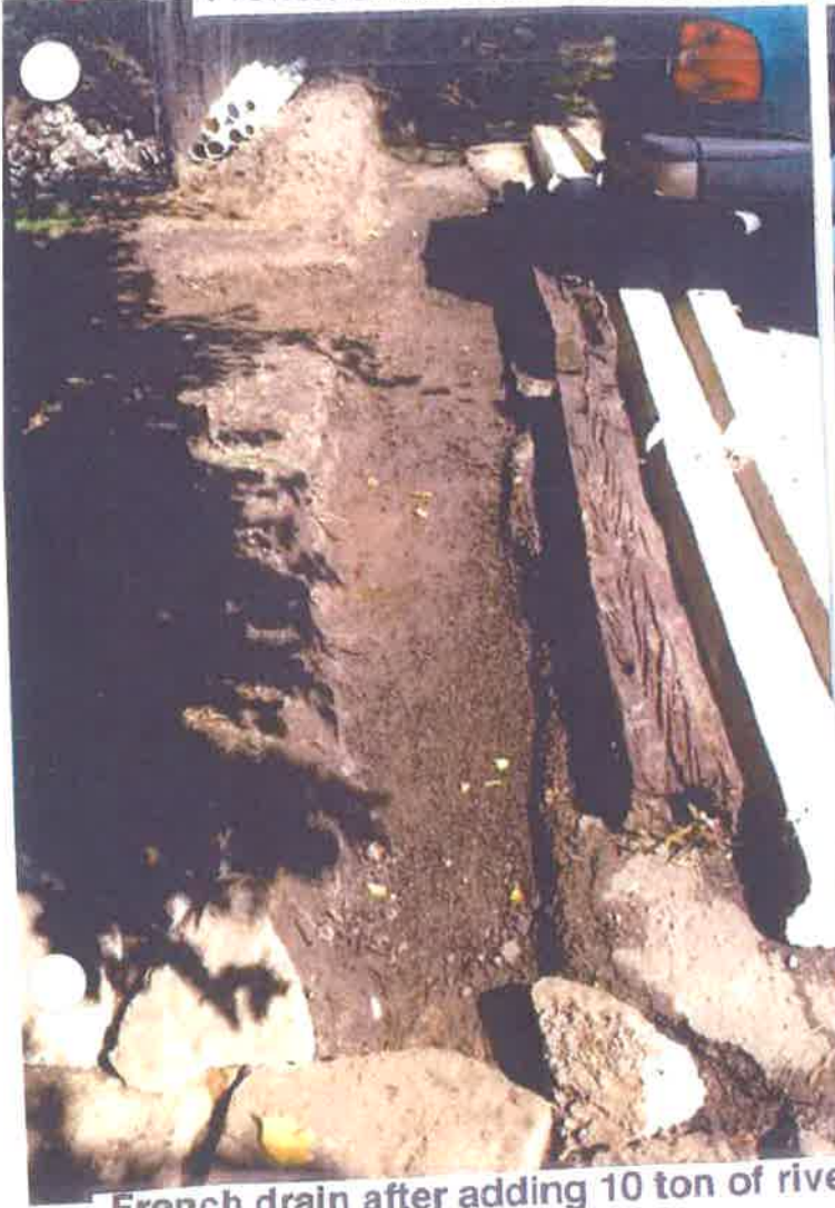
French drain ditch across width of the Right of Way. Note parked truck.
