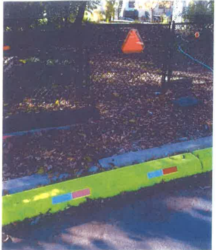
Parking barriers painted with reflective yellow paint and red/white reflective tape Farm implement reflector added to the gate.
