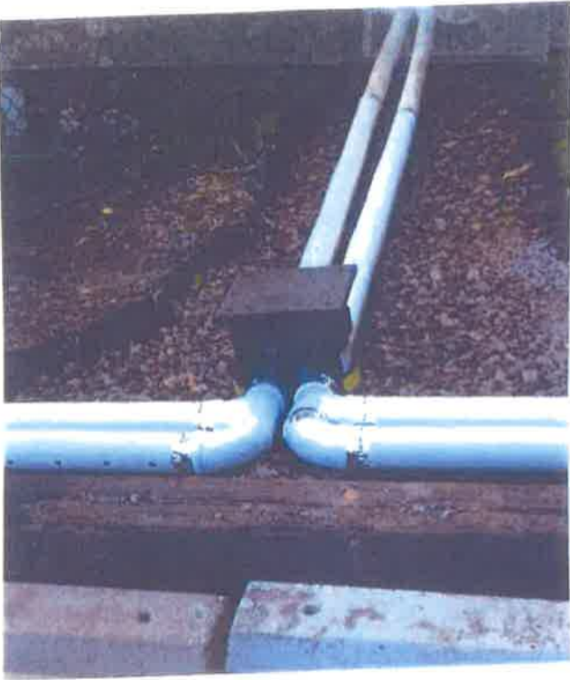
French Drain before covering with river gravel.
