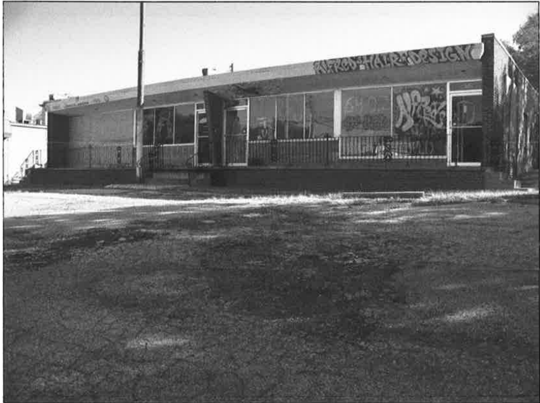
307 NE 58 th Street – looking south – deterioration of parking surface
