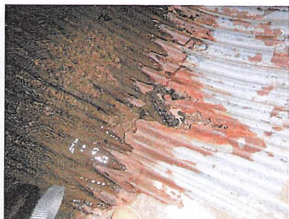
CMP Invert with Rust Holes at 6809 N Agnes Avenue
