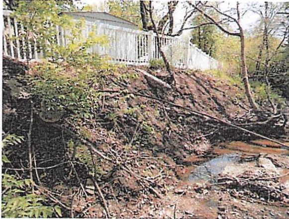
Severe Bank Erosion at 6701 N Agnes Avenue
